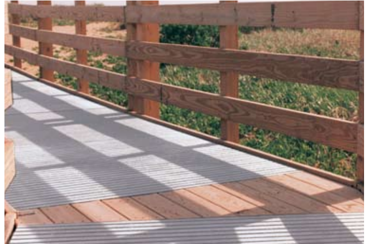
Safe-T-Span pultruded pedestrian grating was chosen for this walkway bridge for swimmers at South Cape Beach State Park near the Cape Cod region of Massachusetts.
