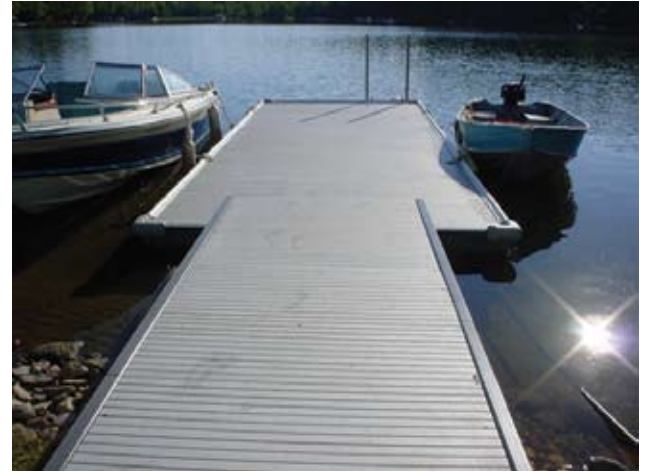
Boat Dock on Horseshoe Lake in Haliburton, Ontario. Safe-T-Span Pultruded Aqua Grate Pedestrian Grating
