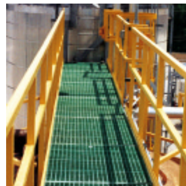
Elevated walkway - molded grating & handrail
